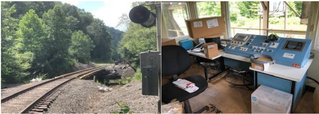
Figure 1: Rail bridge completed; new electrical controls in loadout installed.
